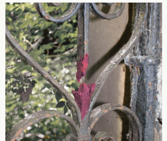
Evidence of two uprising water leaves branching from central stem with corrosion wastage resulting from the water trap they created.
