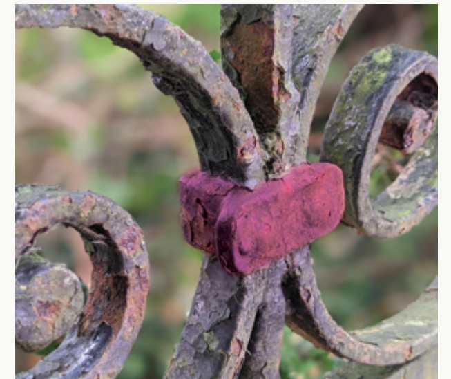
U shaped collar joined with a flat bar riveted in place is characteristic 18 th C cold fitting technique.
