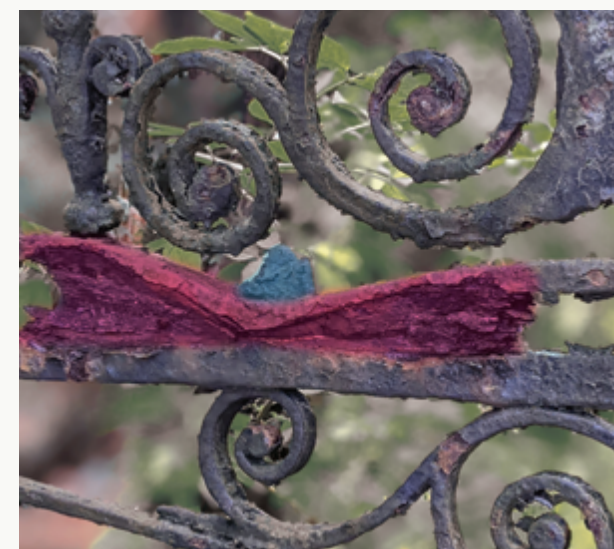
Typical 18th C wedge joint (blue) holding overthrow to stretcher frame, distorted by rust heave as a result of crevice corrosion.
