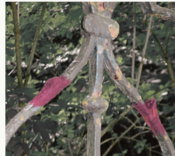
Stubs evidence missing components above fire welded branch joints.
